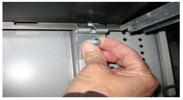
Screw into place using self tapping screws included.
